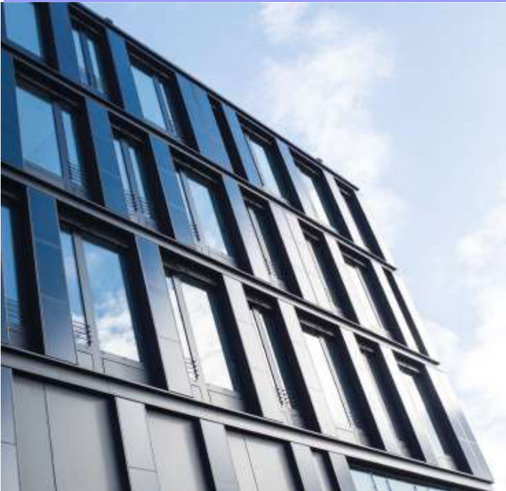
The ZSW institute's building in Stuttgart-Vaihingen has a façade with CIGS panels.
